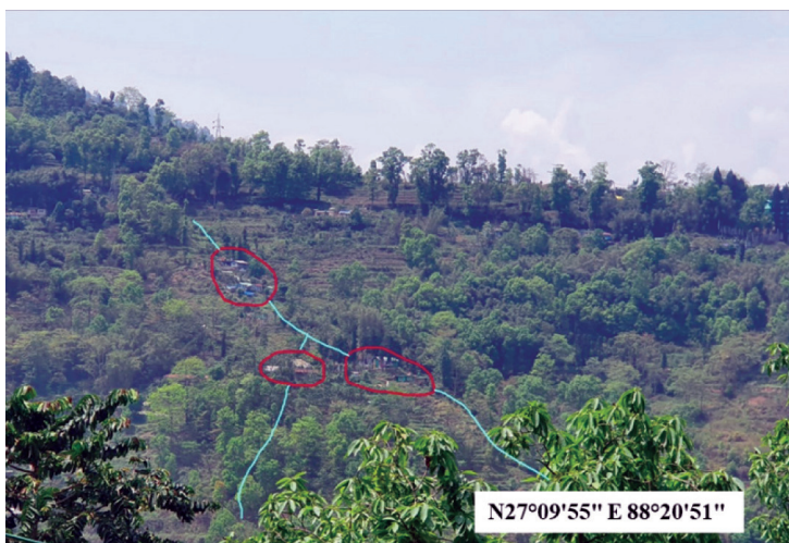
Figure 13. Settlements obstructing the natural stream flow near Namchi have impeded the stream's course, leading to increased seepage and subsequent soil creep in the area.
