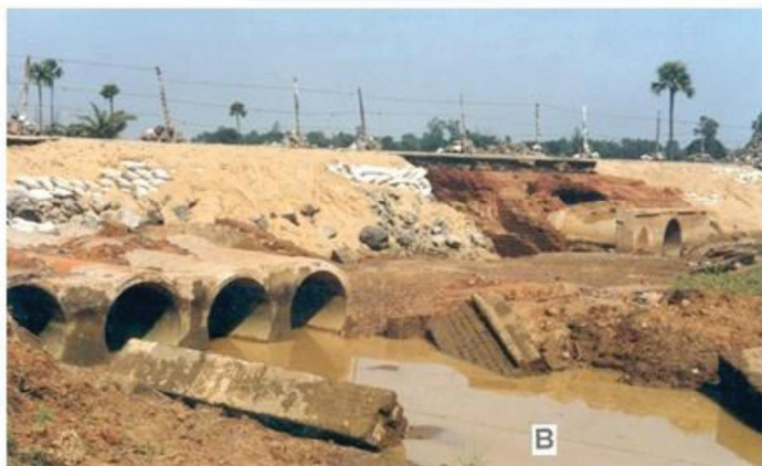
Figure 3. Rejuvenation of Bidya nala (BN) around Satkahania (S) Ajoy River (AR) during high flood; causing severe damage to the Panagarh-Moregram Expressway, 2000. A) IRS Satellite Image (Base of the image: 24.10 km; Central coordinates: 23°33'35" N and 87°36'36" E); B) and C) Field photographs showing ground reality.
