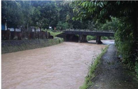
Plate 3. Monsoon flow with high suspended sediment load near Rongtong Bridge
