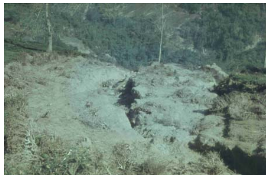
Photo 4. Shallow sliding and piping in Bannockburn (October 1968)
