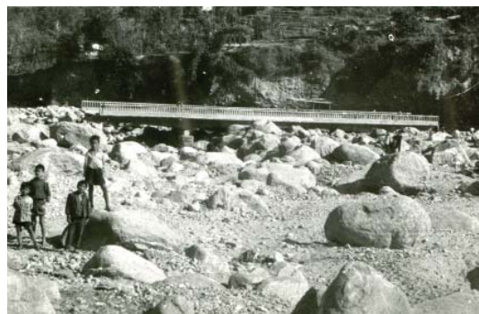
Photo 6. Aggradation of 10 m at the Pool-Bazar bridge (October 1968)
