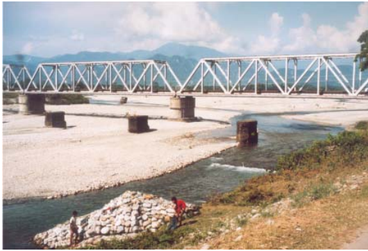
Photo 19. Aggradation of the Chel river bed following subsidence in the piedmont, where a new bridge is constructed
