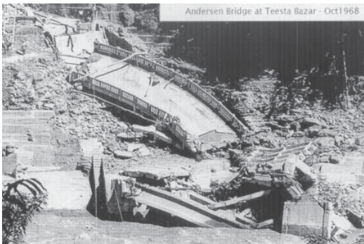
Photo 15. Breaking of the Tista bridge at Tista Bazar in 1968
