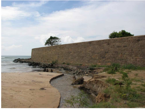
Fig. 23. The high wall of the 18th Century Vattakottai Fort.
