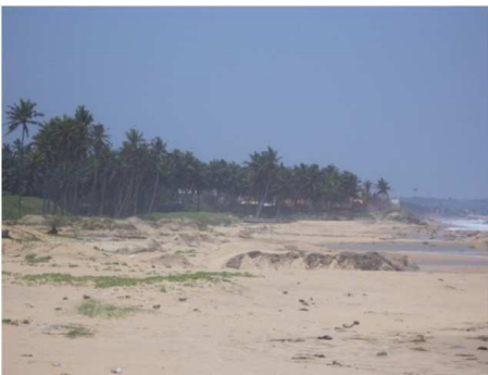
Fig. 33. Coastal erosion between Kanyakumari and Kovalam.
