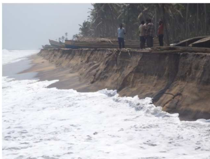
Fig. 42. Beach erosion at the Midalam coast.
